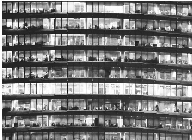
Many office buildings in Asia still blaze brightly all night, but easy-to-use 'eco-switch' systems can make a big difference in energy costs.
